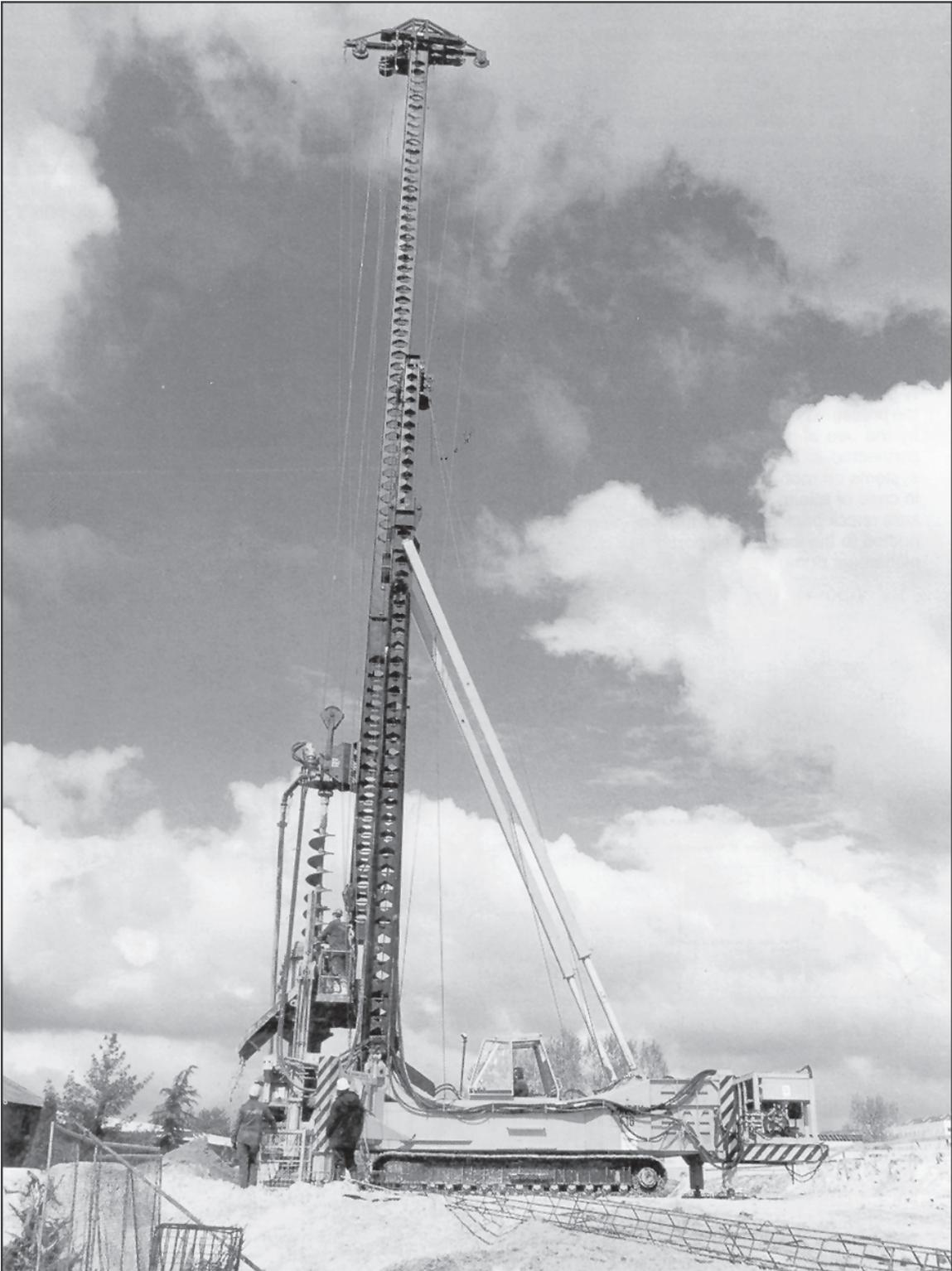
Fig. 23 Hydraulic foundation rig
