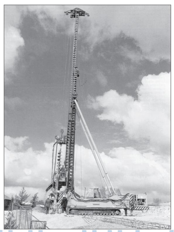
Fig. 23 Hydraulic foundation rig
